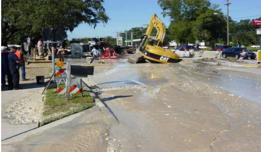
Figure 1 The site of an excavator hitting a utility line
