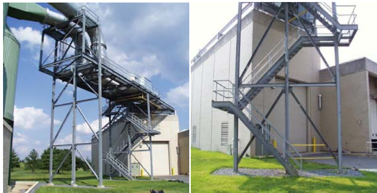
Figure 6: Steel Structure on NIST Main Campus
