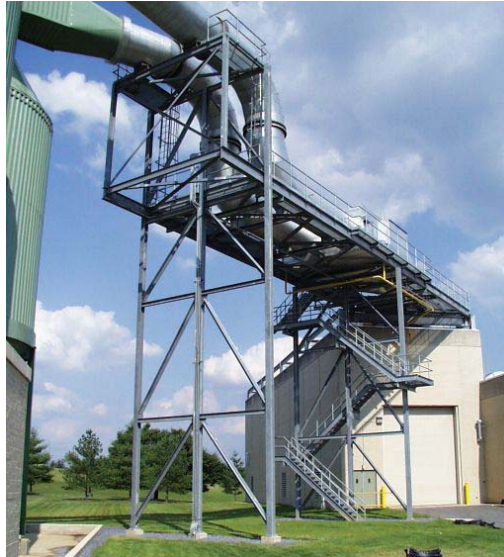
Figure 4 – Steel Structure on NIST Main Campus
