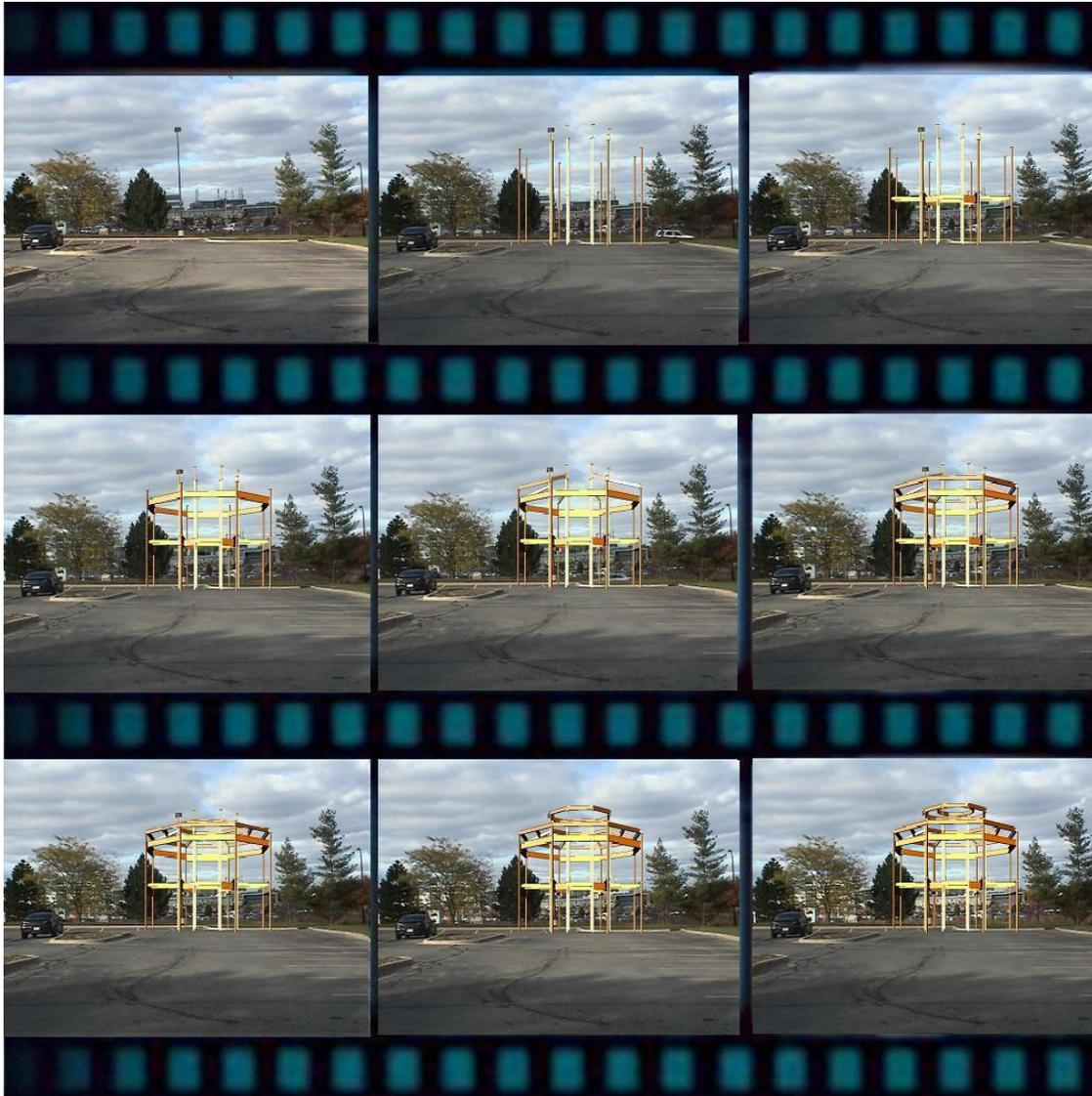
Figure 3: Augmented reality visualization of a steel structure erection operation
