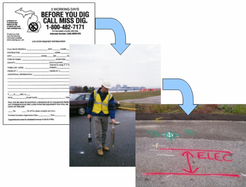
Figure 1 – Process of Manually Marking the Underground Utility Lines
