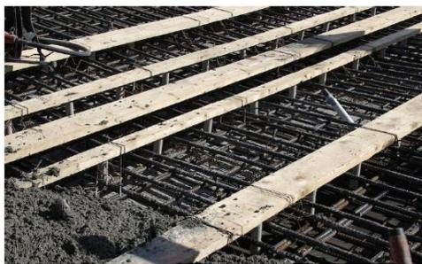
**Figure 1: A railway bridge deck rebar cage with the dowels and wooden planks installed [Saidi, K., et al., 2011].**
